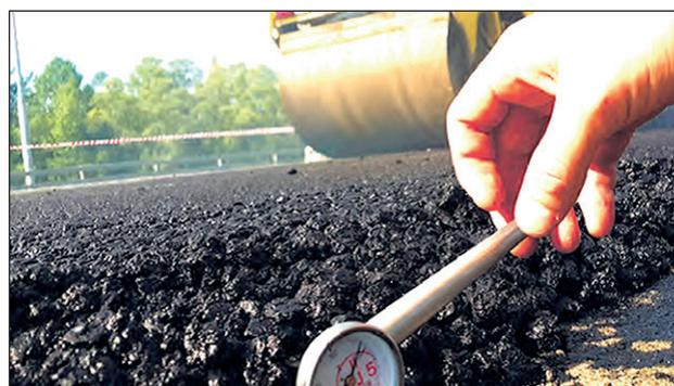
Fig. 5. Control of asphalt concrete roadway laying using polymer-bitumen nanocompositions
