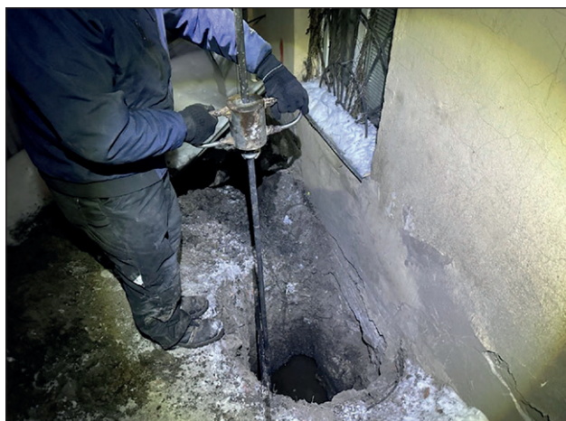
Fig. 7. Investigation of the properties of stabilized soil using the probing method
