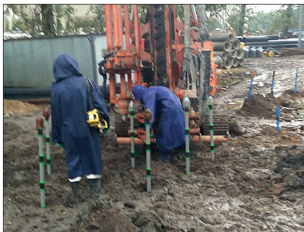
Fig. 2. Soil stabilization by injection (collar technology) – injector installation shown
