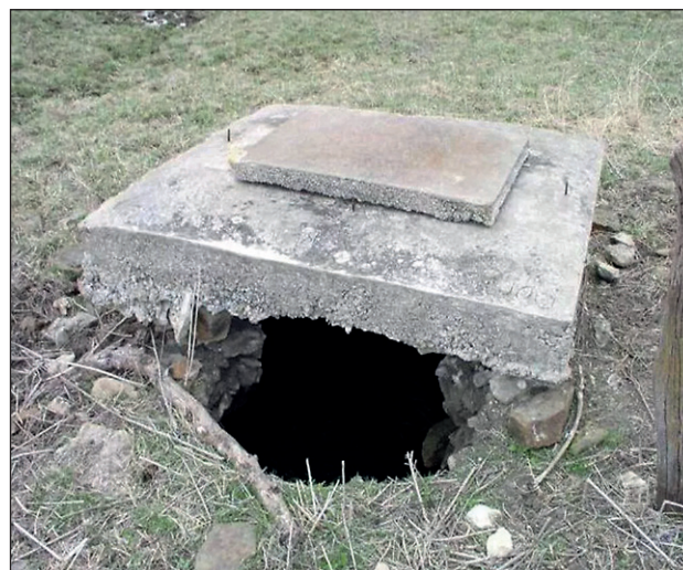
Fig. 3. Consequences of well abandonment according to the “standard design”
