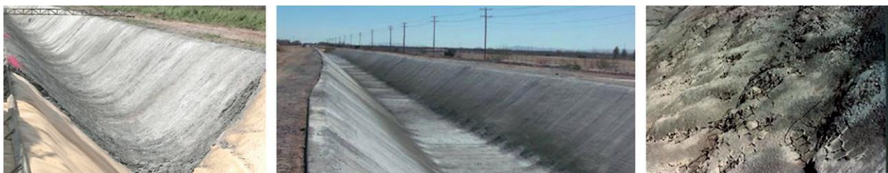
Fig. 1. Pilot sites of irrigation channel lining installation using shotcrete in the south of Kazakhstan
