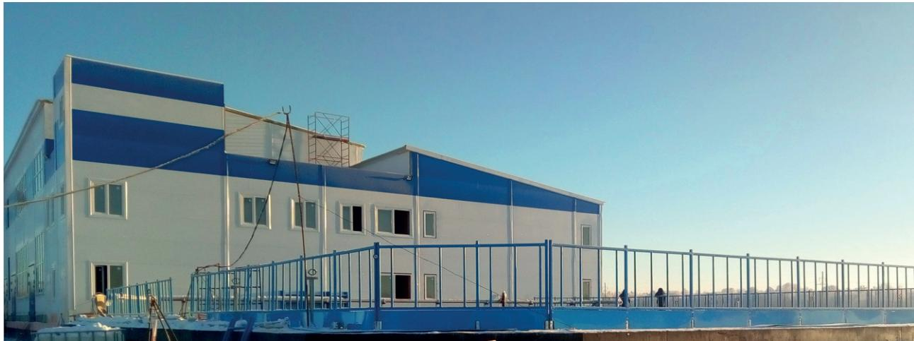
«**N**anotechnological center of composites» («NCC») which stockholder is Fund of infrastructural and educational programs by RUSNANO developed and launched production of special composite handrails made of glass-fiber composite. The pilot project has been performed on poultry plant «Yaroslavsky broiler» (Yaroslavl) in the course of modernization of aerotanks of waste treatment facilities.
