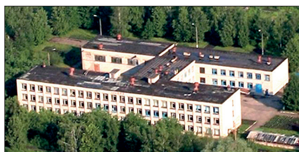
Fig. 4. School building according to the standard project 65-426/1 for 960 students
